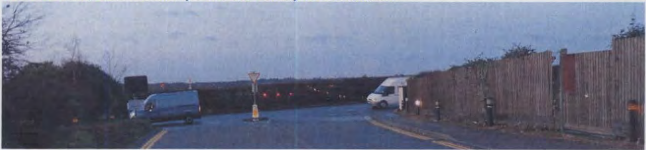
West End Road, Eastern Boundary Fence and Runway viewed from East
