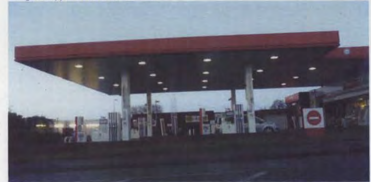
Garage Canopy on A4180 West End Road
