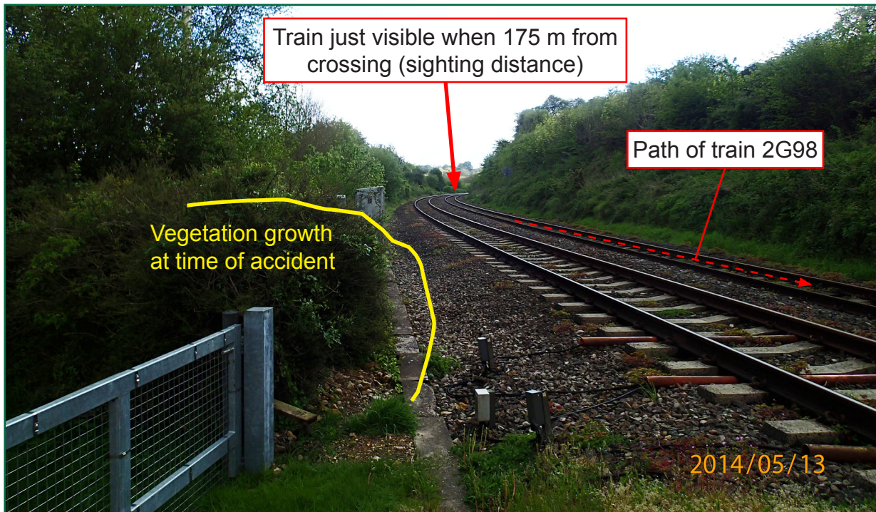
Figure 5: View from north side of crossing towards trains approaching from Swindon (May 2014 photograph)
