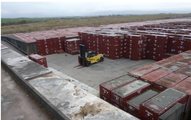
Radioactive waste disposal containers in Vault 8 at LLWR, courtesy of LLW Repository Ltd
