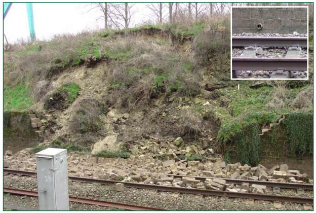
Figure 4: Derailment site showing cutting slips, state of backfill and typical weep hole (inset)
