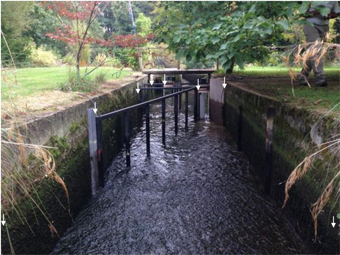
Figure 3.2 Photograph of the screen installation and bypass (to left and downstream of the screen) along with hydrophones in place (flow direction is going away from the camera). Note the screens are not in place in this photograph and the flume has been de-watered. Experimental water levels are indicated by the high water line on the bypass deflector. White arrows indicate approximate location of hydrophones
