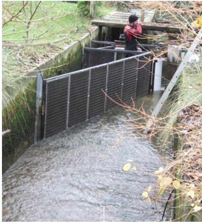
Figure 3.3 Photograph with screens in place. Note the flume has been de-watered in the photograph
