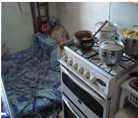
Figure 3.4: Dwelling with a higher than average risk of fire and harm from flames and hot surfaces
