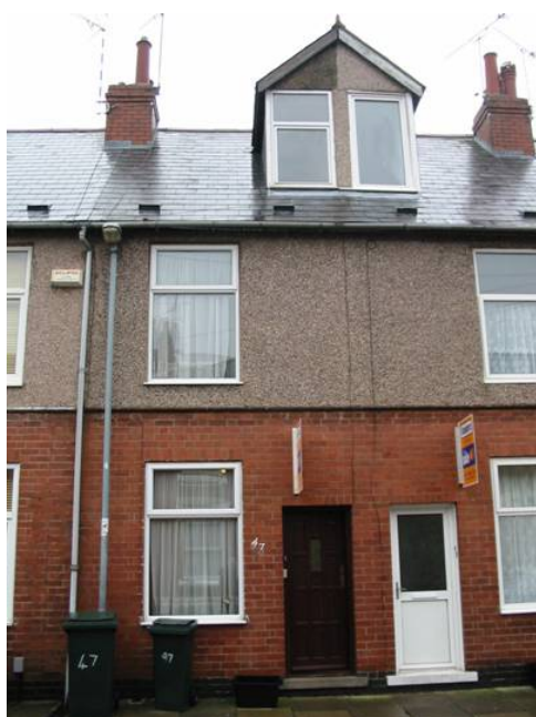
Figure 3.6: Example of a mid-terrace property with a Category 1 fire risk
