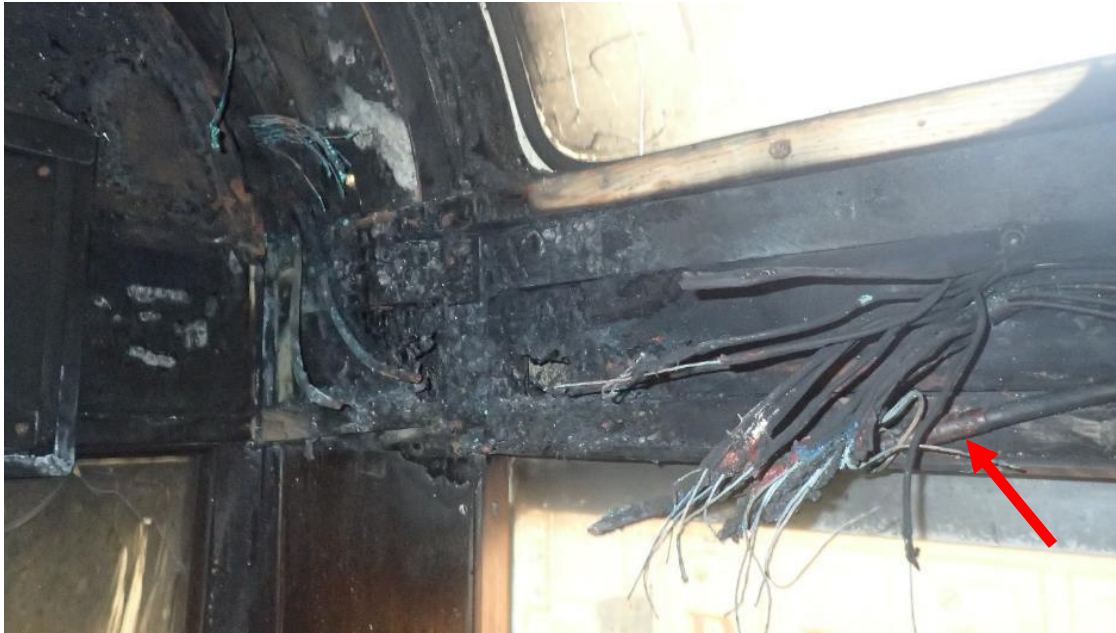
Fire damaged cabling within 272; the previous cable repair is indicated by the arrow
