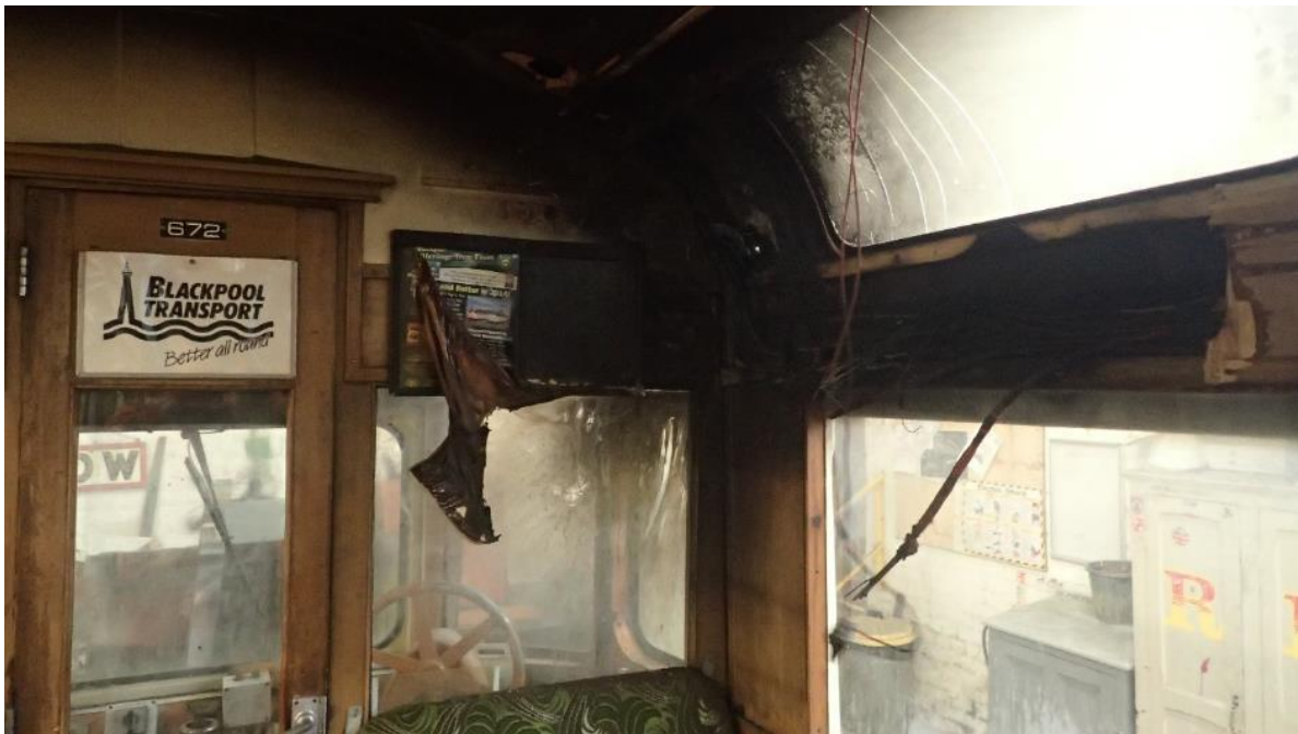
Internal damage to 272
