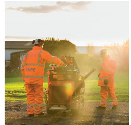
Ground investigation is key to the early construction programme.
