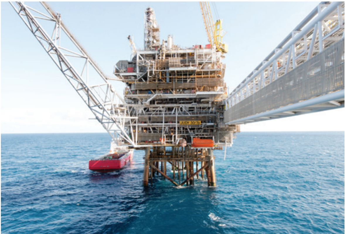
The Judy Platform and Bridge Link to the Judy Riser Platform
