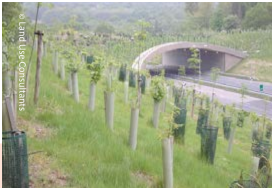
A21 Scotney Bridge following construction (2005)
