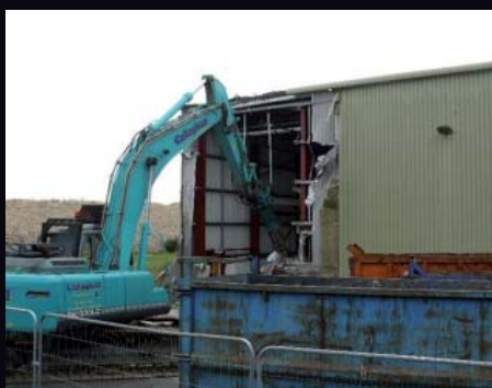
Demolition work under way at the Waste Encapsulation Treatment Plant
