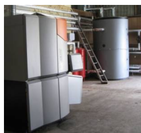
Fig 48 – Biomass boiler
