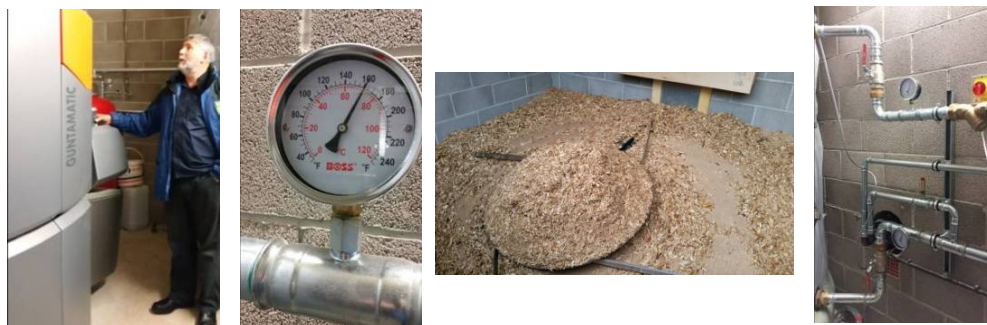
Figs 8 – Guntamatic biomass boiler installed at Dewlands Farm, currently taking woodchip fuel
