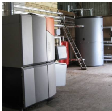
Fig 5- Typical Biomass Boiler
