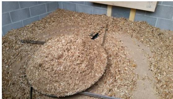
Fig 95– Feed-table for biomass boiler (woodchip shown)
