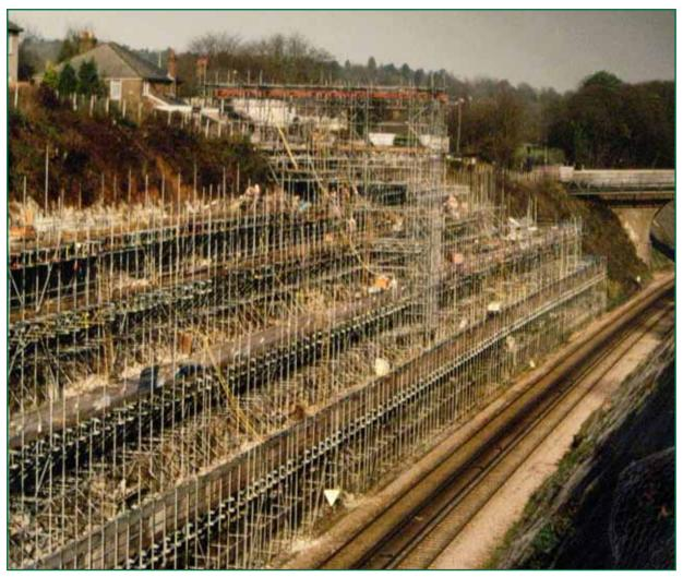
Figure 15: Photograph showing the stabilisation works of 2001 - 3 (courtesy of Network Rail)
