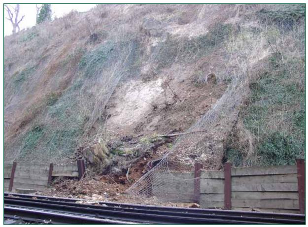
Figure 9: Hooley cutting showing the landslip
