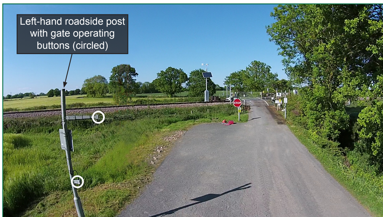
Figure 4: The approach to the crossing towards Oakwood Farm showing the left-hand roadside post
