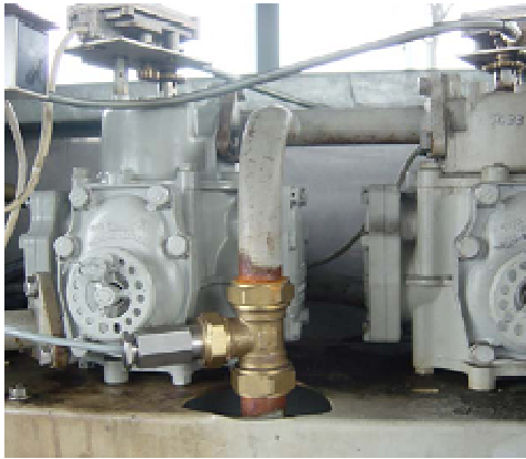
Figure 60 Typical installation of temperature sensor
