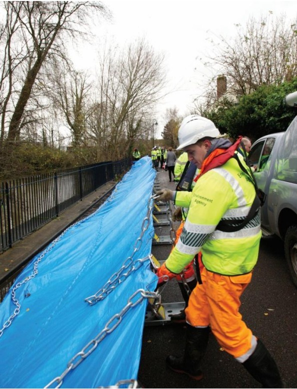
Operations staff installing a demountable defence and carrying out river maintenance in Oxford
