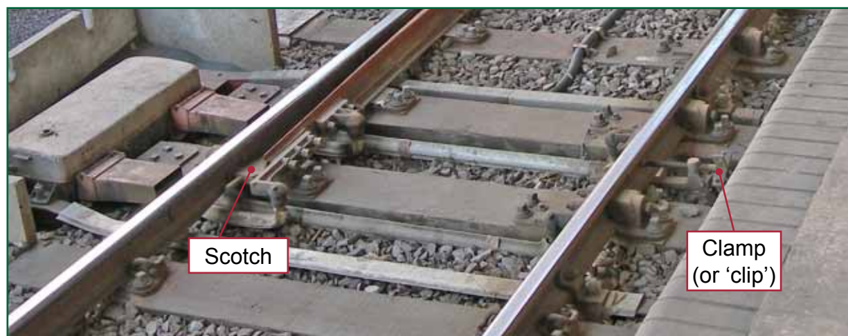
Figure 6: The S&C clipped and scotched out of use
