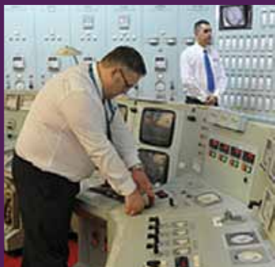
Andrew Freeman has the honour of closing down Oldbury's reactor
