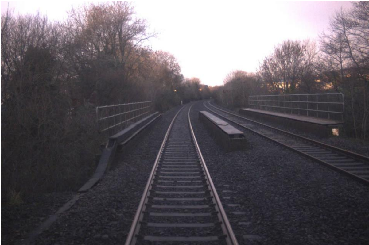
Library image of Maesyfelin bridge (courtesy Network Rail)
