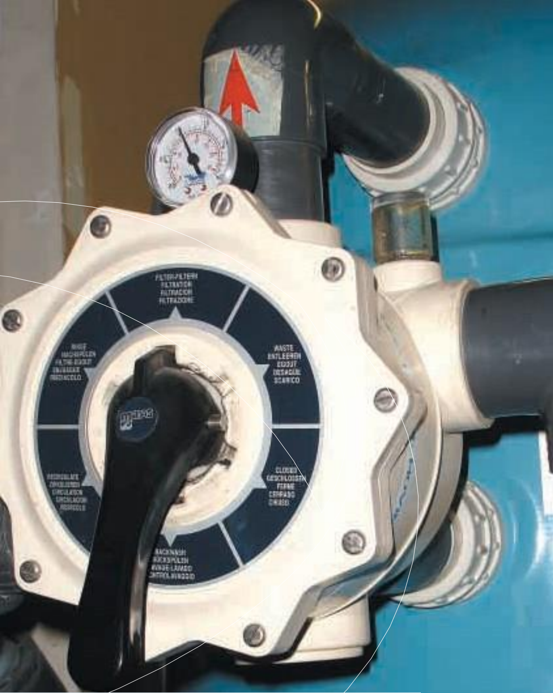
Filter backwash control valve – note sight glass to observe backwash (with kind assistance of Esporta Ltd)
