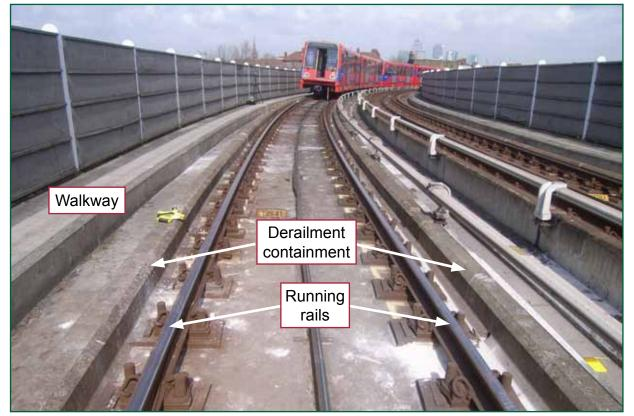
Figure 3: The Lewisham extension showing running rails and concrete derailment containment
