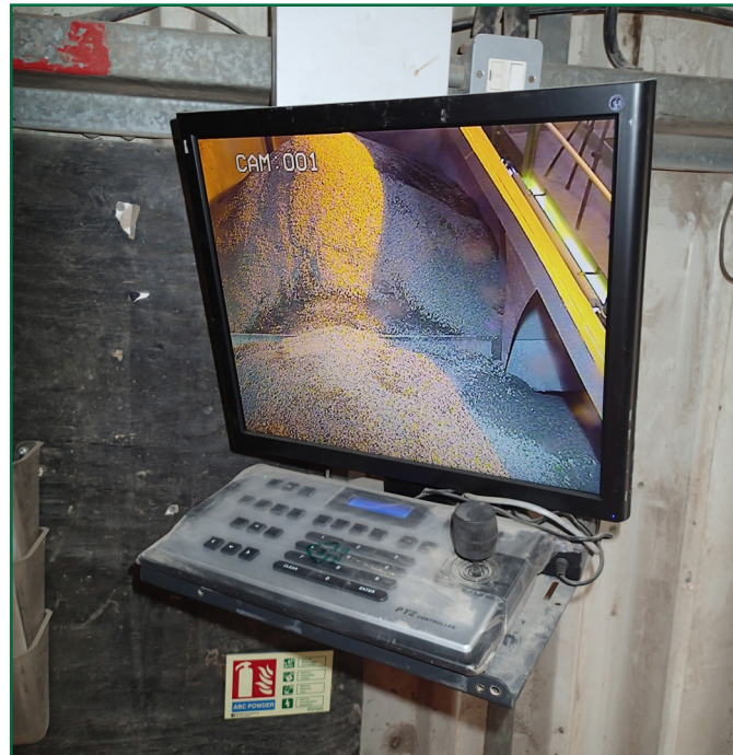
Figure 19: Operators view of wagon interior on CCTV screen
