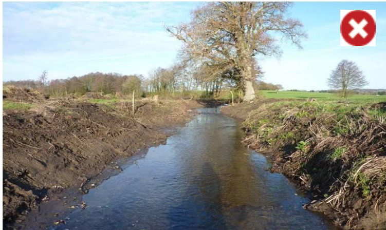
Figure 3: Do not remove the fringe of vegetation or leave watercourse banks bare or exposed like this.
