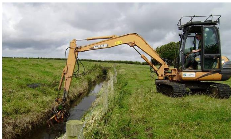
Figure 4: Use an appropriate sized machine and bucket
