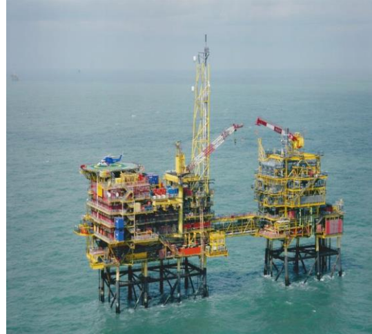
Picture 2: Sean PP & PD installation
