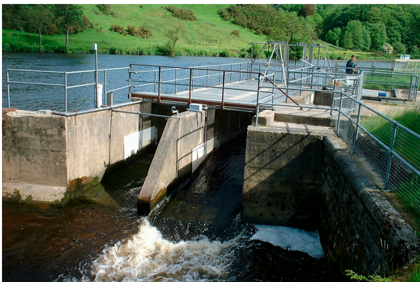
Forge Weir fish trap and counter on the River Lune (photo courtesy of the Environment Agency).
