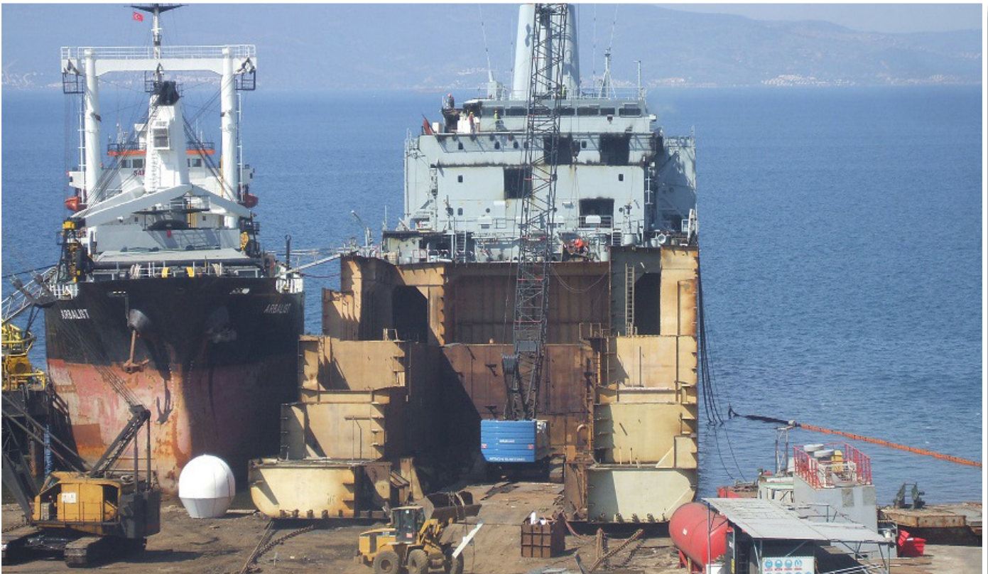
Dismantling and progress of works dated 13 April 2016.
