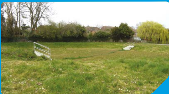
A new SUDS scheme in Leamington. This scheme uses land at the back of a school to collect surface water.
