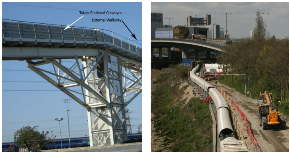
Figure 3.22 Conveyor support structure - left, adjacent vehicle access (Crossrail) - right
