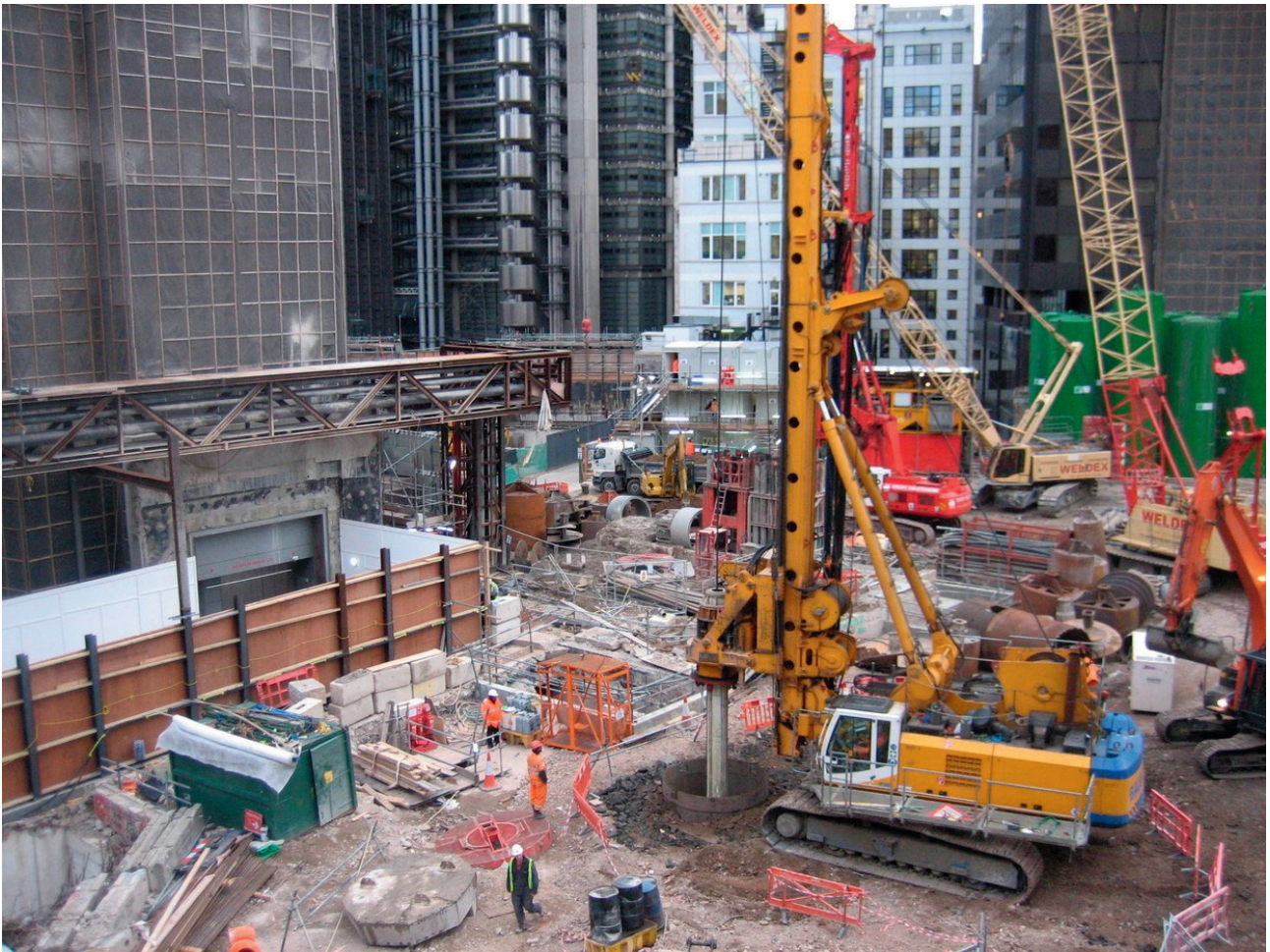
Figure 20: Photograph of an example of a piling rig
