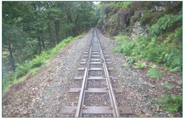
Figure 4: Ffestiniog railway track without baseplates, as originally fitted at Gysgfa
