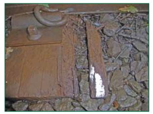
Figure 8: Timber sleeper affected by decay
