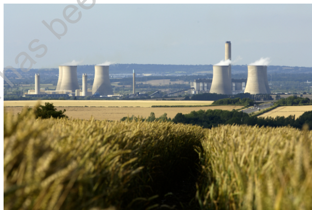
Figure 2 – This image shows Didcot A, a dual fired power station which used tower cooling when operational. It closed in March 2013
