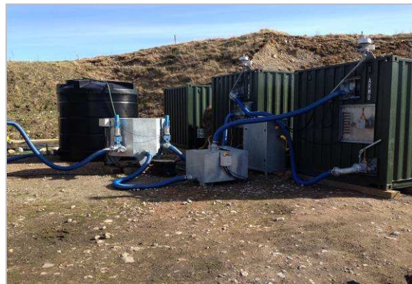
Figure 10: Connection from settling tanks located in screw press module to reception hopper which then feeds into the anaerobic digester
