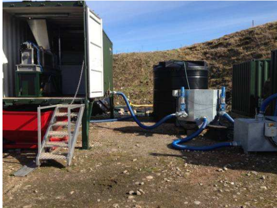
Figure 10: Connection from settling tanks located in screw press module to reception hopper which then feeds into the anaerobic digester
