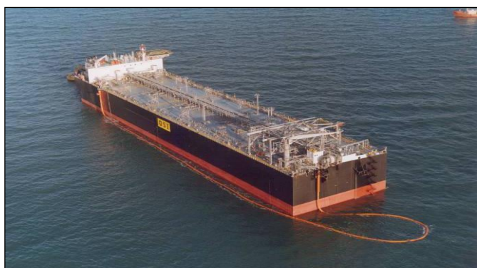
Photo 4 - Oil Storage Installation
