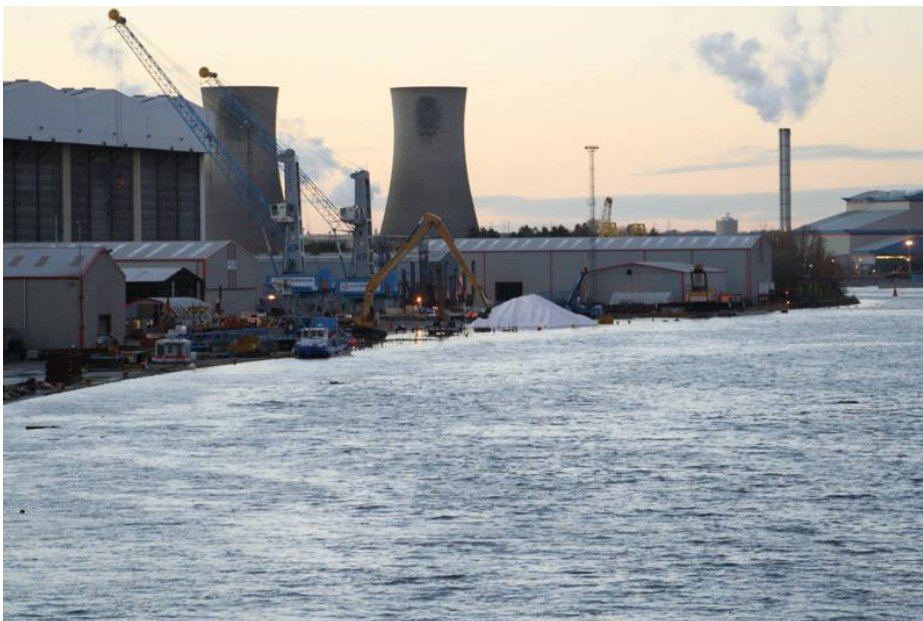
Figure 2. Dawson's Quay showing the very high water levels during the 2013 tidal surge (image PD Teesport).
