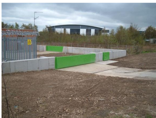
Substation sites protected by a bund wall with gate access
