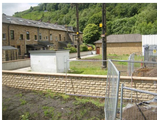
Bund wall under construction
