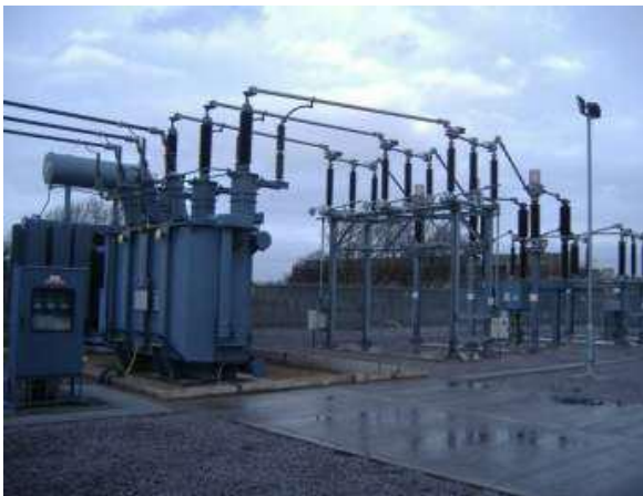
Figure 3 - 132kV Grid Transformer and Circuit Breaker in service in the UK
