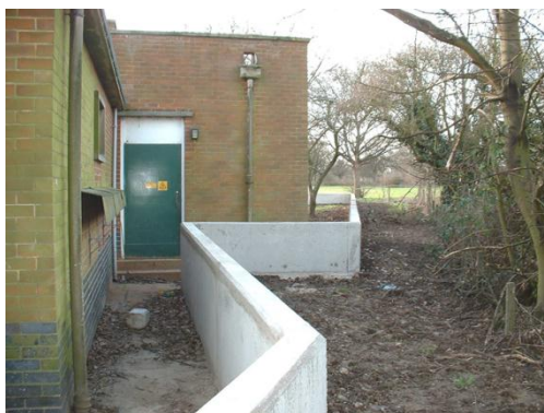
Substation sites protected by a bund wall with gate access
