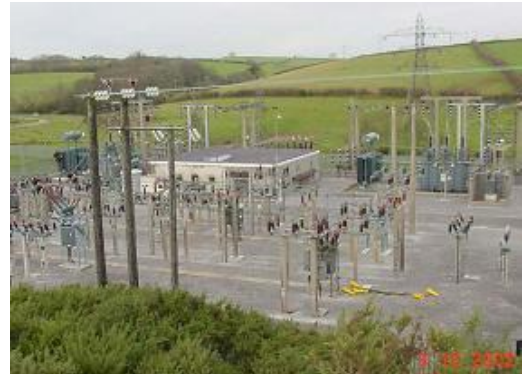
Figure 16 - 132kV Grid substation showing 132kV terminal tower and start of 33kV wood pole overhead line
