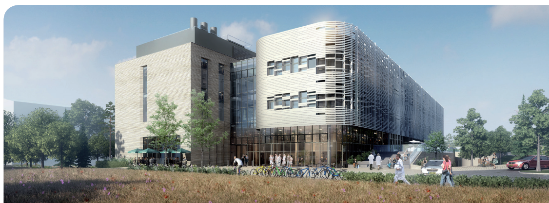
The Quadram Institute – building work started in February on the new centre for food and health research to be located at the heart of the Norwich Research Park, with an anticipated opening in 2018.
