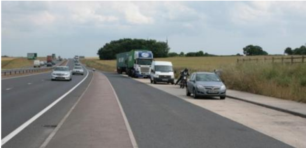
Figure 3-8 – Lay-by on new A14
