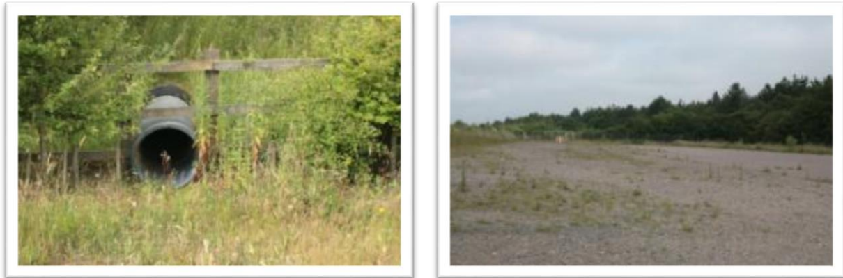
Figure 5-19 – The mammal tunnel exit (left) into the contractors compound (right).
