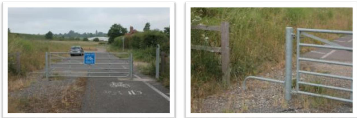
Figure 5-26 – Gate and stile arrangements constituting a trip hazard for horses at the end of the NMU link near Haughley New Street.
