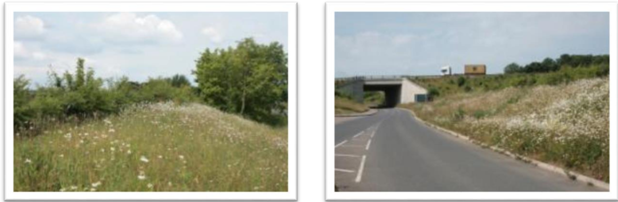
Figure 5-12 – Wildflower planting performing as expected on the new bund adjacent to the old A14 immediately west of Tot Hill Junction (left), and adjacent to the old A14 along the north side of Quarries Cross underpass (right).
