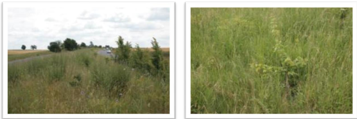
Figure 5-6 – The left picture shows the new bund and planting between the restricted highway (left) and local access road (right); the right picture is representative of the individual plant stations on the bund.
