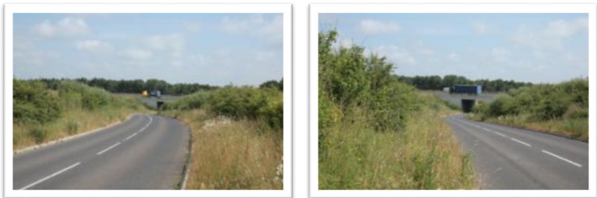
Figure 5-3 – Established planting performing screening function approaching Quarries Cross underpass from the south.
