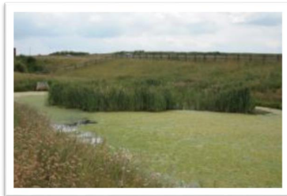
Figure 5-16 – The balancing pond to the east of Tot Hill junction contains a significant quantity of pond weed, but reed and marginal planting is well established.
