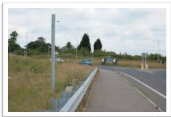
Figure 5-29 – Damaged directional sign adjacent to the footway approaching the northern roundabout at Tot Hill junction from the new overbridge; the mounting post remains in situ (left), with the plate at its base (right).
