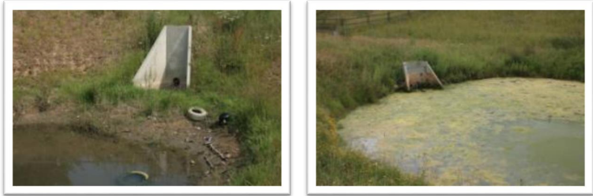
Figure 5-23 – Potential partially blocked inlets/ outlets at the Quarries Cross junction balancing pond (left), and Balancing Pond 3 to the east of Tot Hill junction (right).
