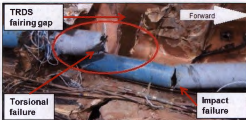
Figure 1.4.32 - Catastrophic torsional failure of No 5 TRDS
