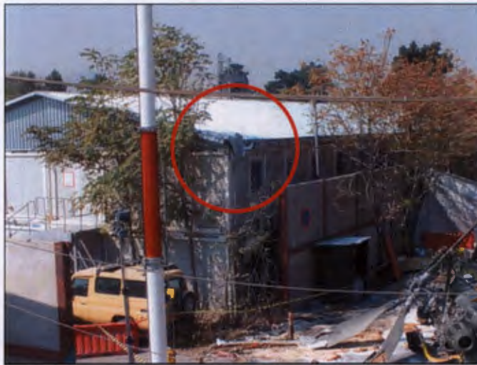
Figure 1.4.35 - Damage caused by MRBs
