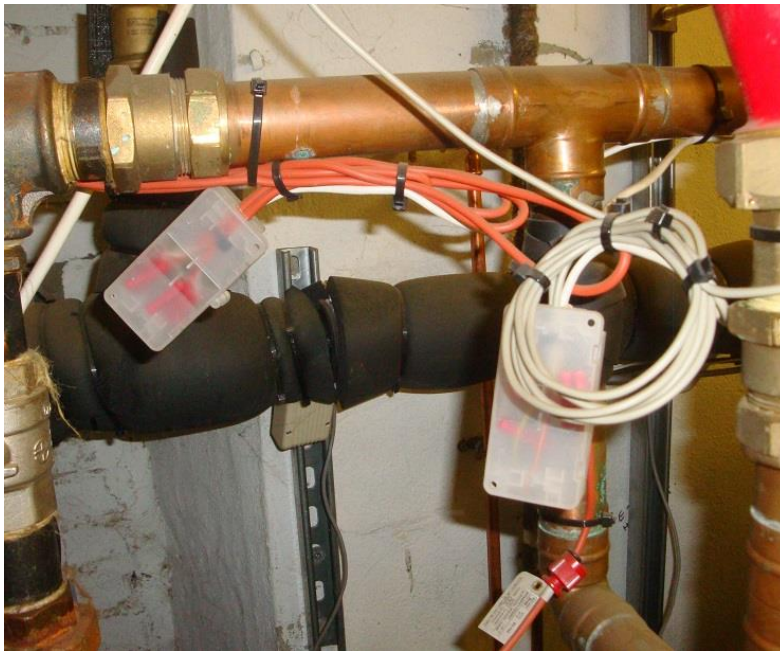
Figure 66 – Temperature sensor leads extended
