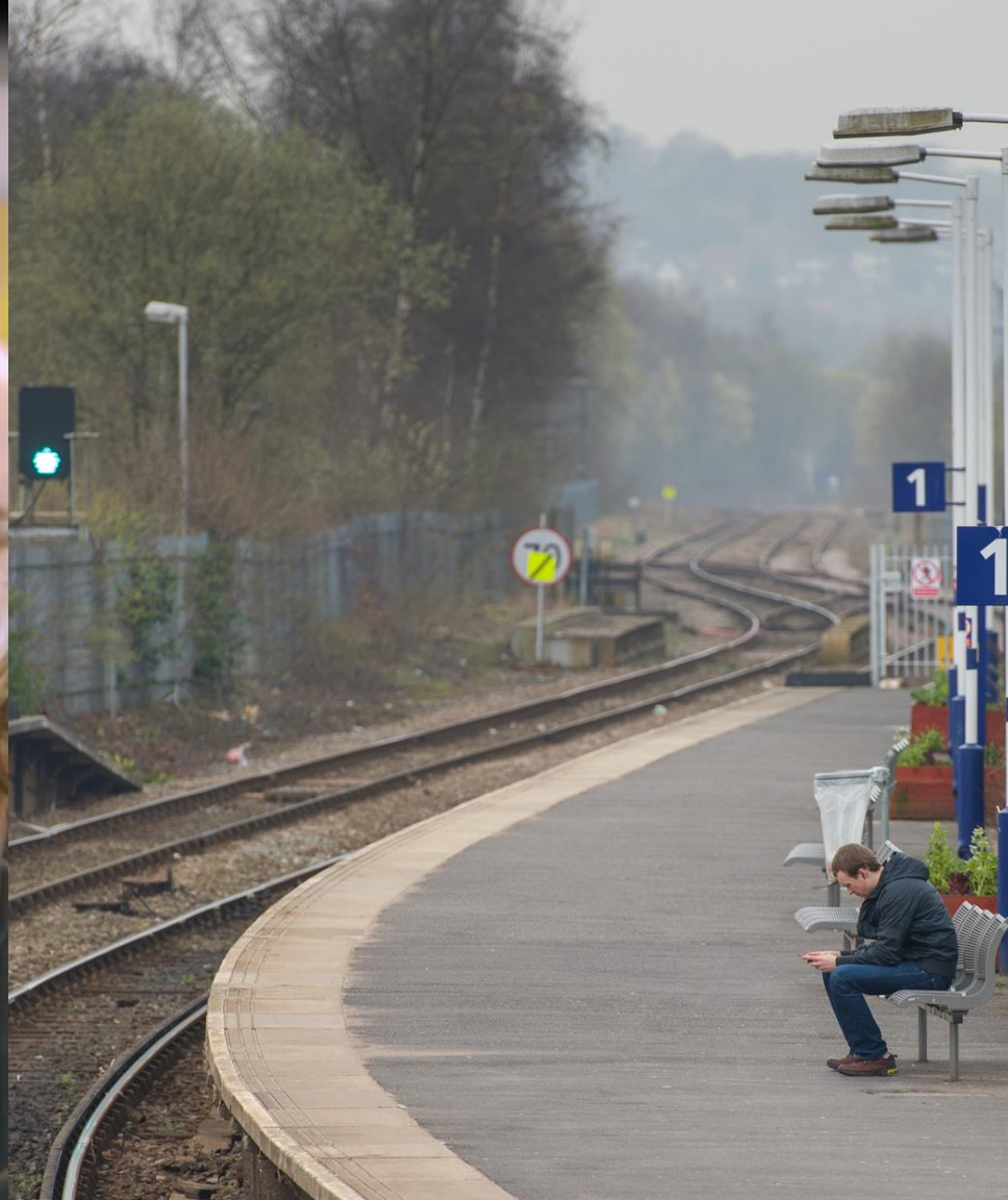
Poor connectivity in the North
