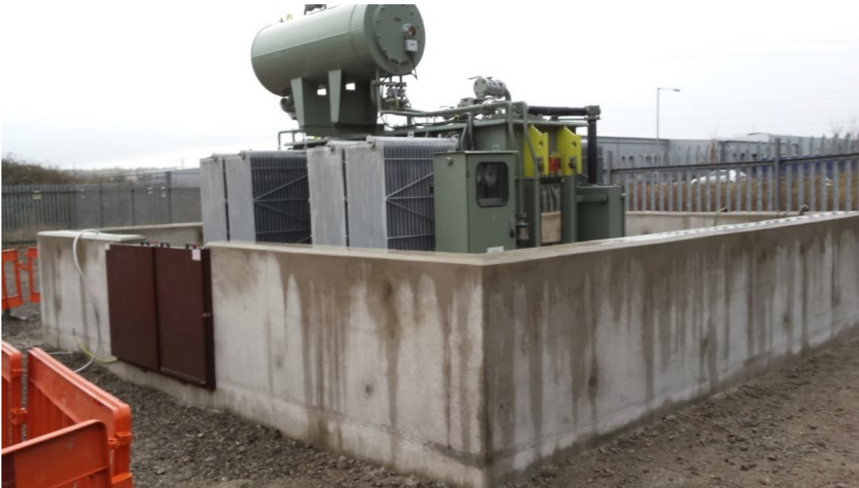
Figure 10.2 Primary Transformer at Queensferry Primary Substation - Height of bund wall increased and flood proof door installed
