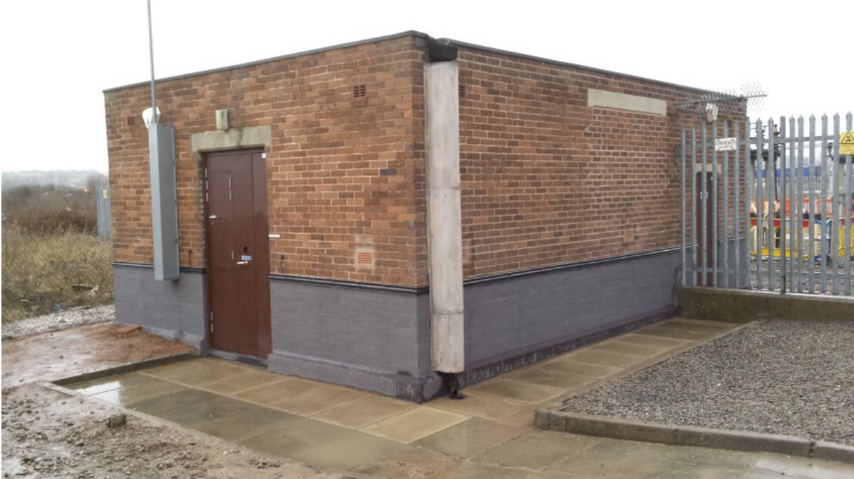
Figure 10.2 Primary Transformer at Queensferry Primary Substation - Height of bund wall increased and flood proof door installed
