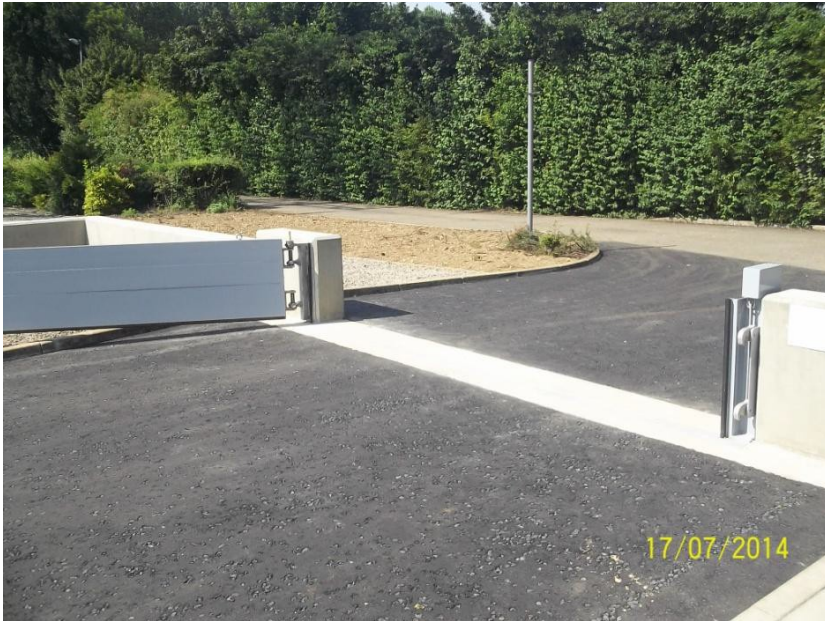
Bund wall and flood gates protecting a site (Courtesy UKPN)
