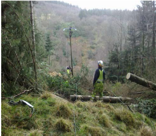
Figure 10.4 Tree damage to overhead line (left) and example of ETR132 tree clearance works (right).
