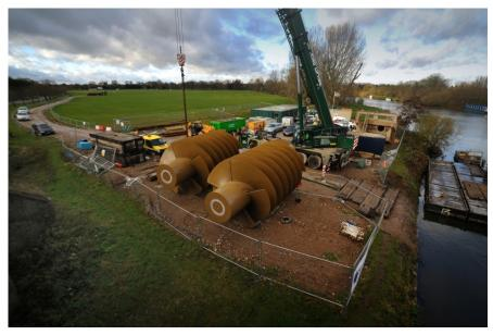
Two 40-tonne Hydropower turbines installed at the Environment Agency's Romney Weir on the River Thames.
