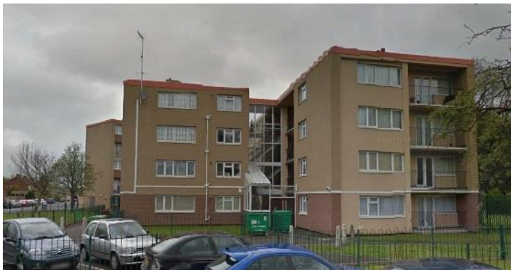
Figure 1 Typical Smaller MDU Henbury Court (Flats 47 – 62)
