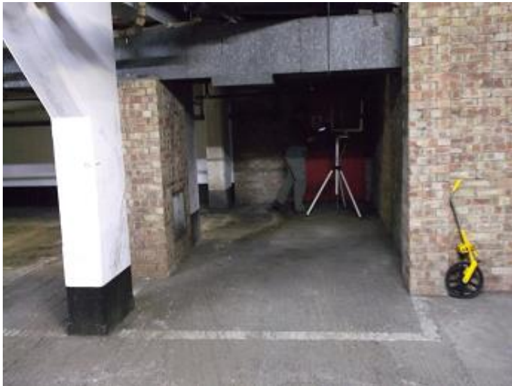
Figure 9 Test Location 2-2 Basement Garage
