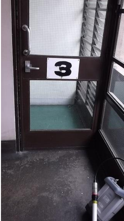
Figure 4 Typical Test Location on the Central Staircase
