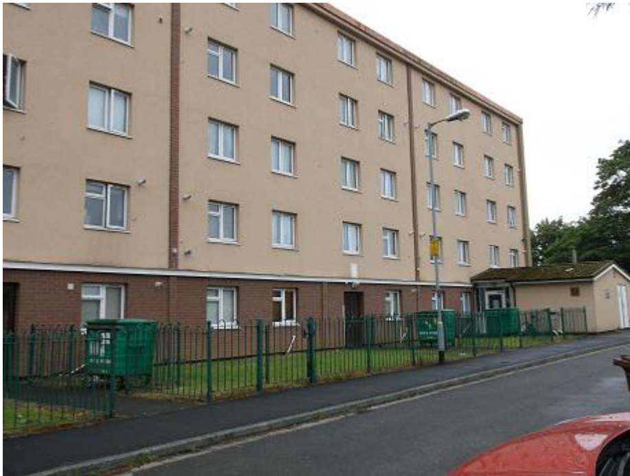
Figure 2 Larger MDU Henbury Court (Flats 1 – 30)
