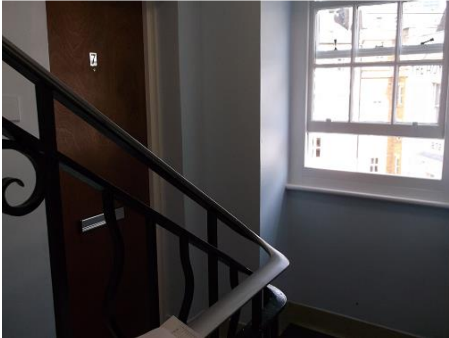
Figure 5 Test Location 1-1 Landing outside Flats 7 and 8
