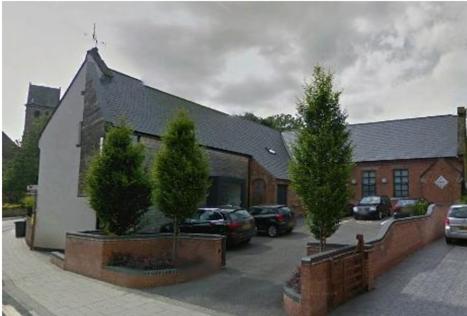
Figure 1 Typical View Michon Creative Building
