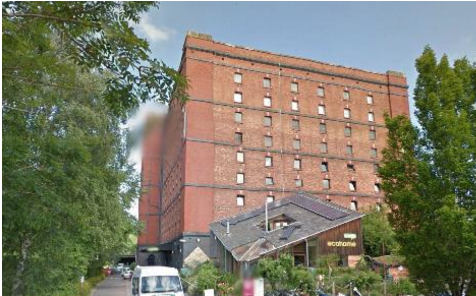
Figure 1 Typical View 'B' Bond Warehouse
