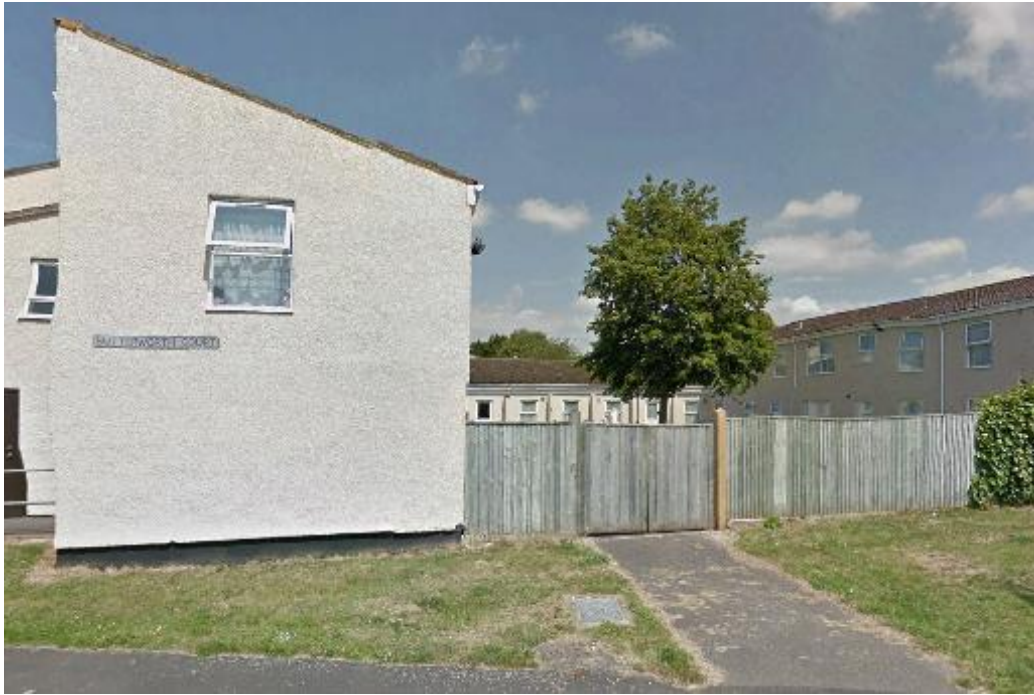
Figure 1 Typical View Butterworth Court
