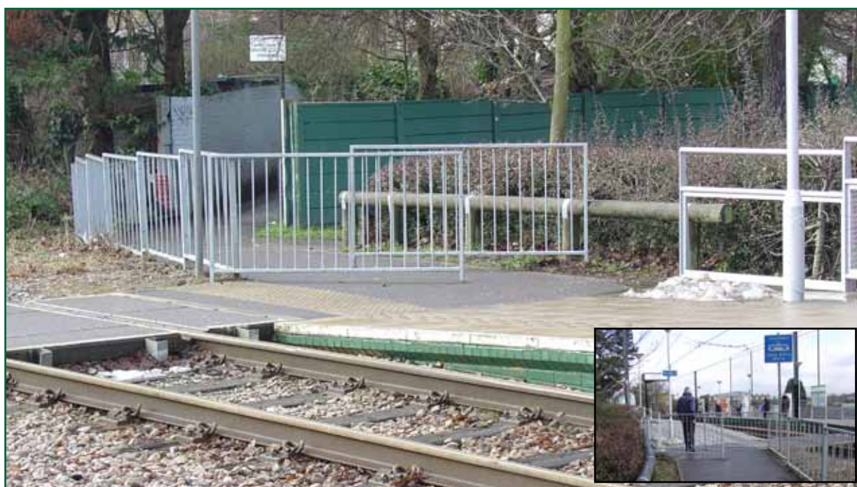
Figure 7: Chicane installed at Arena tram stop
