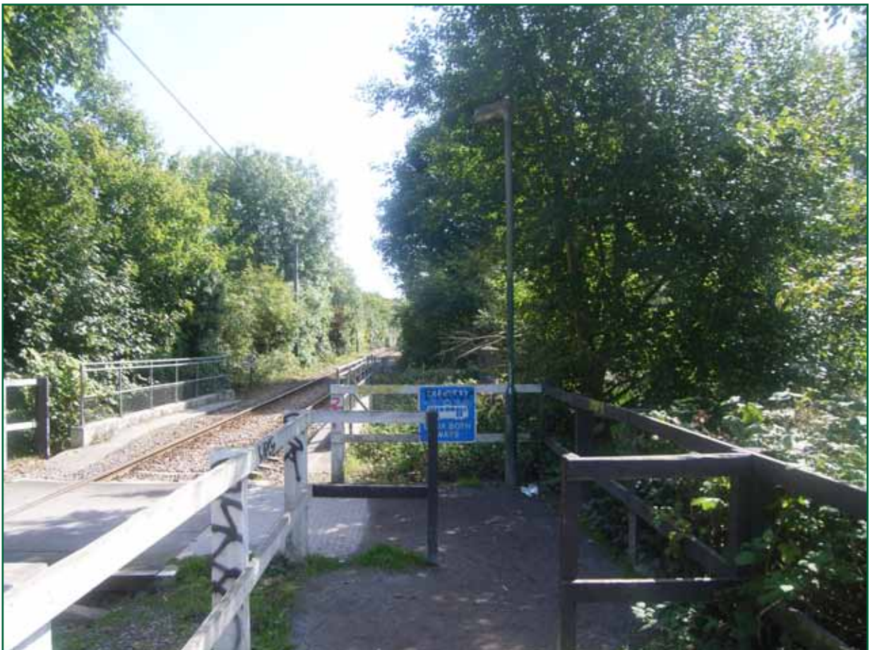
Figure 6: View towards Phipps Bridge, south-east from crossing
