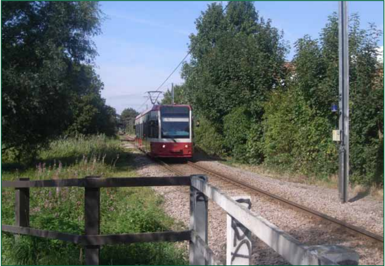
Figure 5: View towards Morden Road, north-west from crossing
