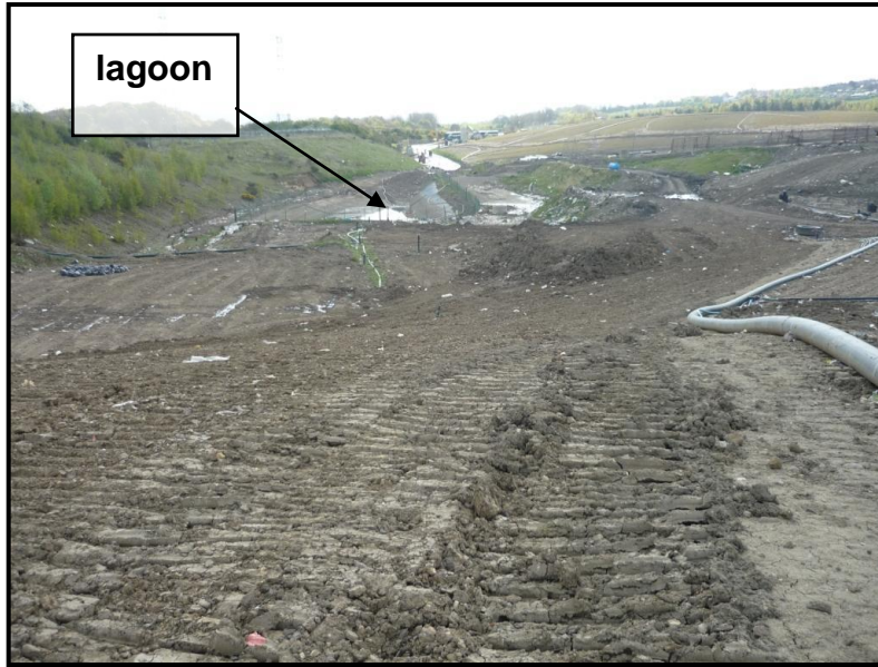
Clay capped area of cell 3 – looking east towards site lagoon and Hexham Old Road
