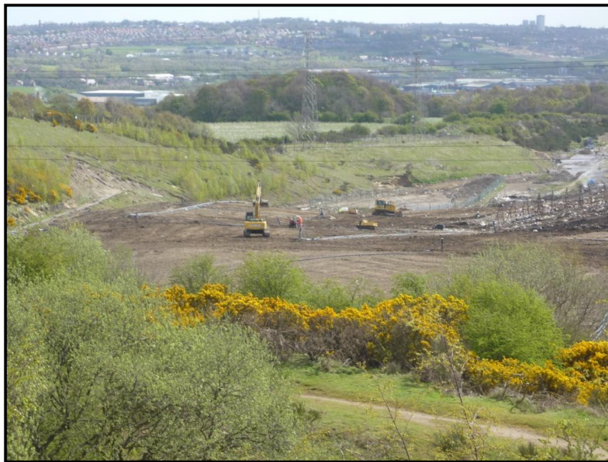
Clay capping work being undertaken (looking from Stargate)
