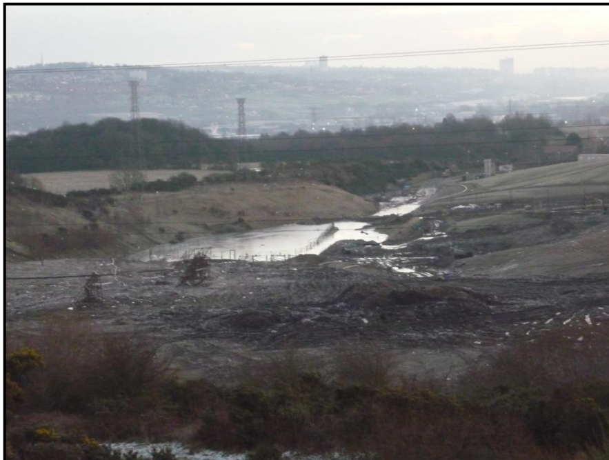
Flooded lagoon from cell 3 – looking east (January)
