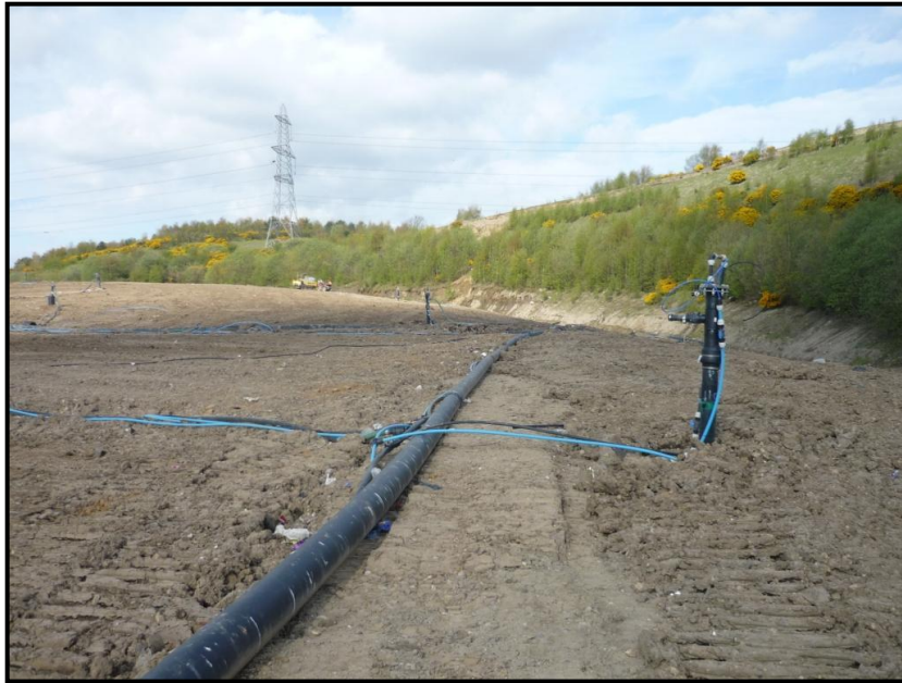
Clay capped area of cell 3 – looking northwest towards the ‘mound’
