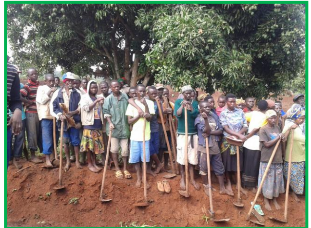
Public Works beneficiaries of a terracing project in Mugesera Sector during a field visit to the DFID-supported Vision 2020 Umurenge Programme (VUP) in Eastern Province
