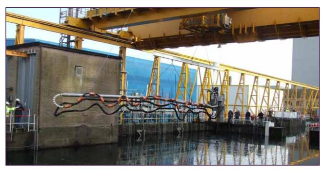
The Sludge Retrieval Hood in operation at the open air pond
