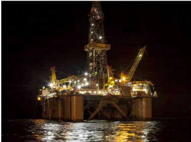
Figure 2.11 WilPhoenix Drilling Rig
