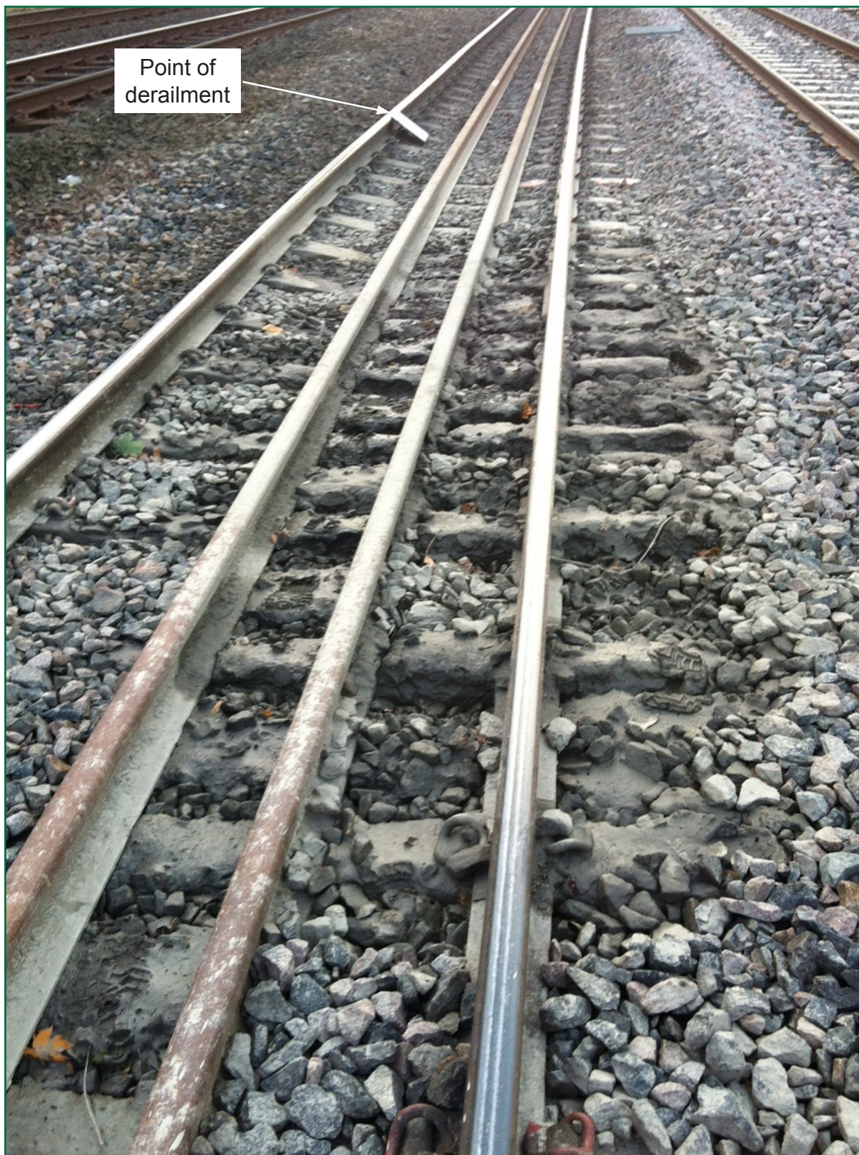
Figure 19: The ballast and wet beds on the approach to the point of derailment (image courtesy of Network Rail)
