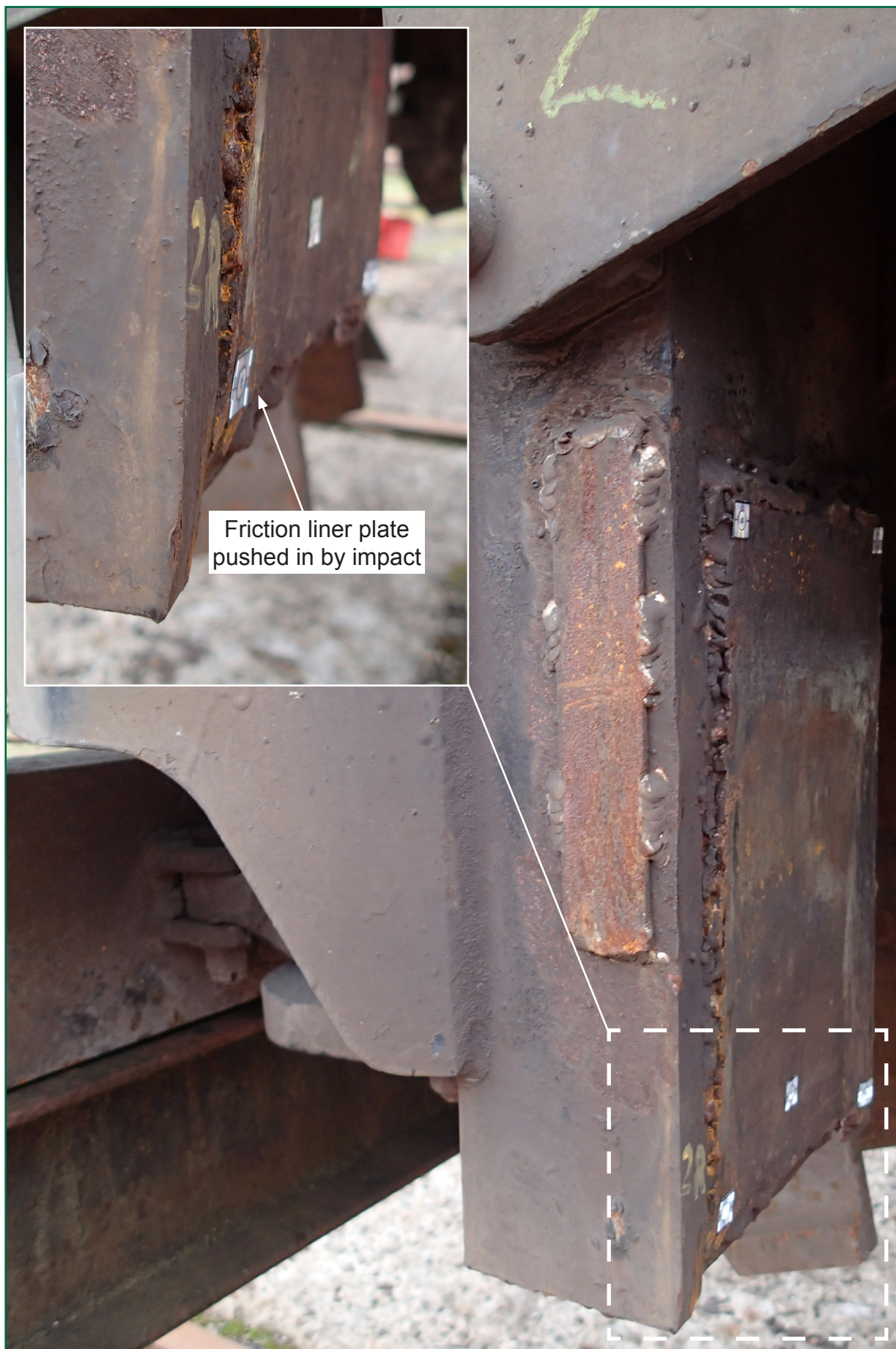
Figure 16: The damage to the trailing right-hand pedestal
