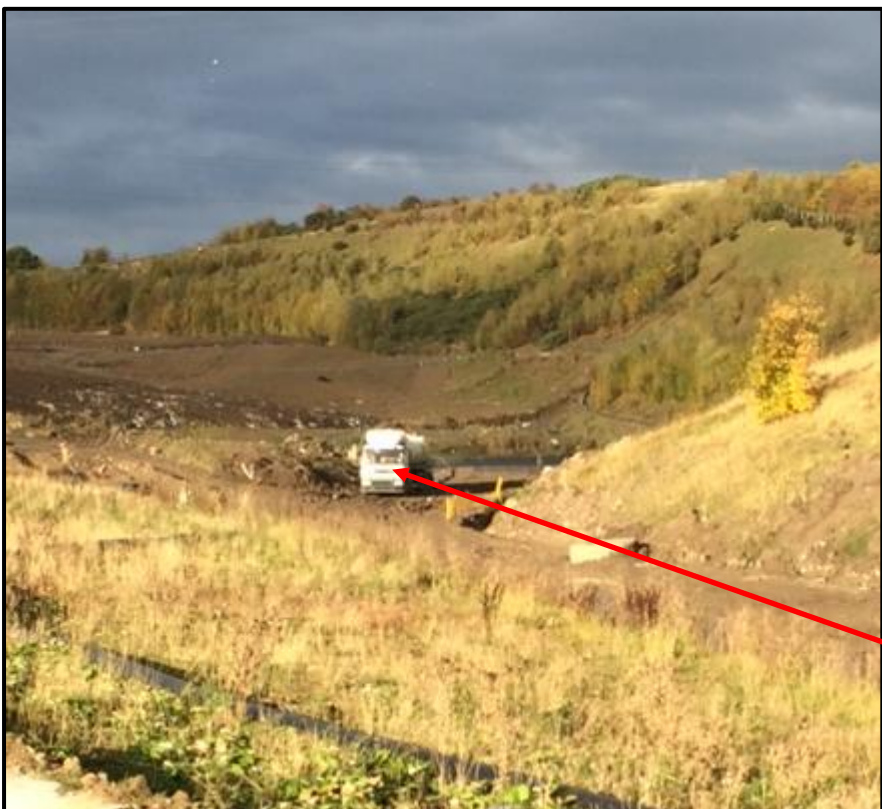
Tanker removing water from surface water lagoon
