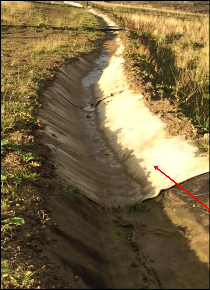
Surface water drainage ditch
